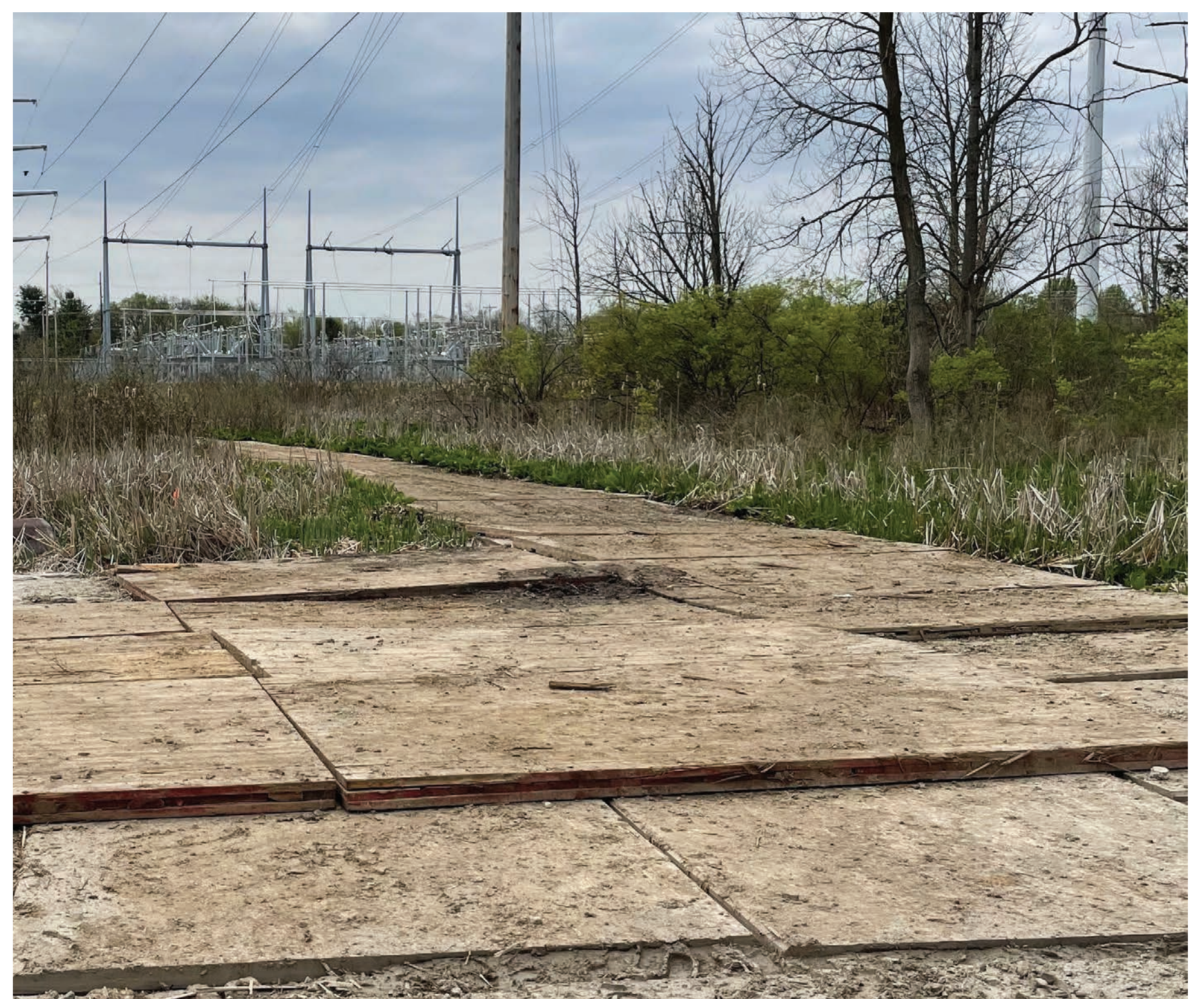
Construction mats minimize erosion of soil during construction and restoration of work areas.
