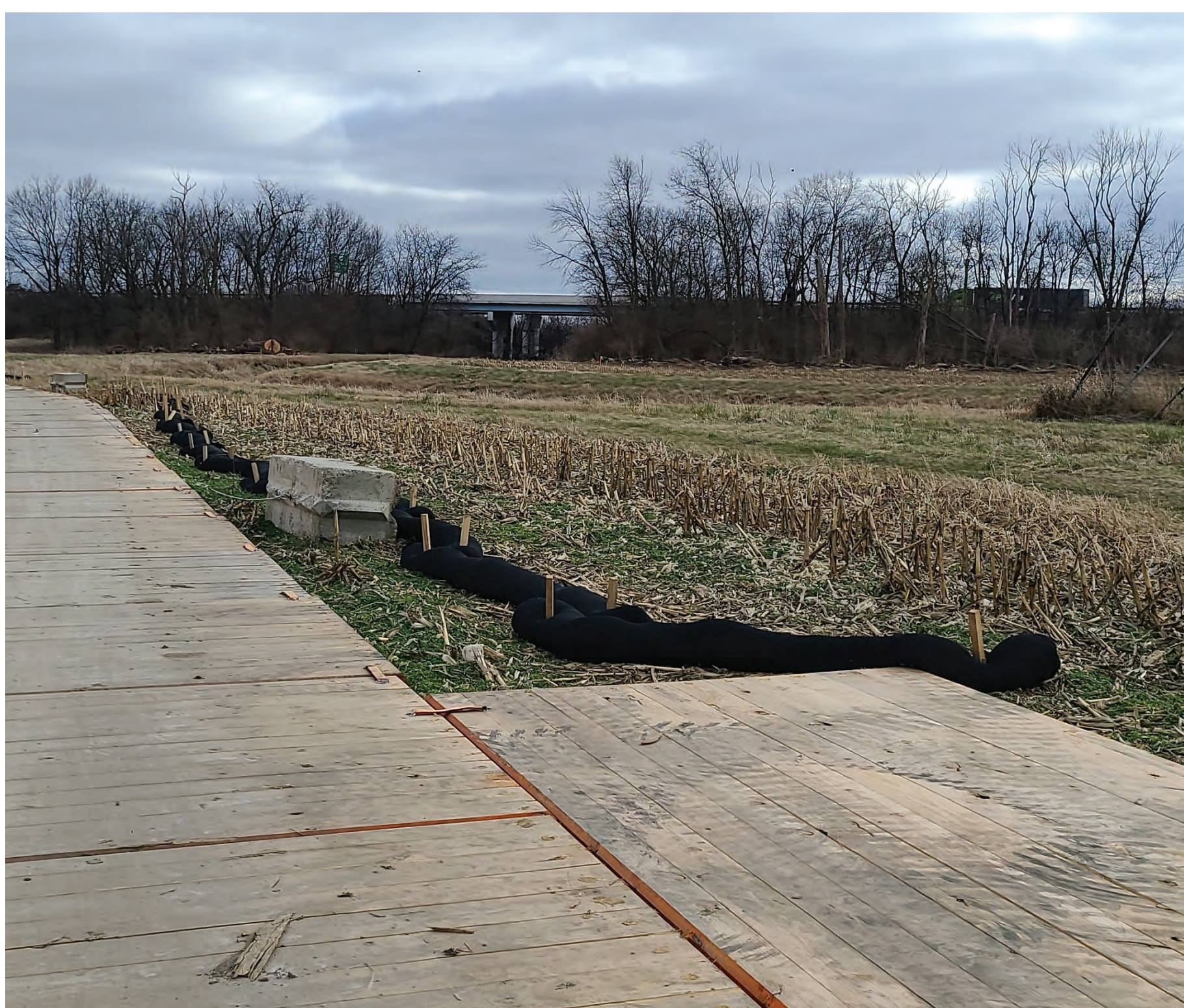
Filter socks and construction mats limit soil erosion and protect streams and rivers.
